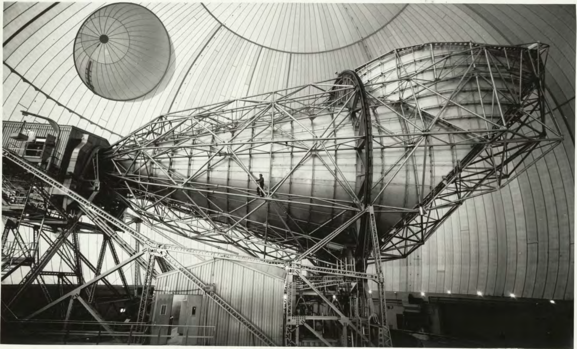
Giant 340-ton antenna inside radome. Housing at left holds maser and other gear enabling antenna to send signals up to satellite and receive faint signals sent back to earth.
